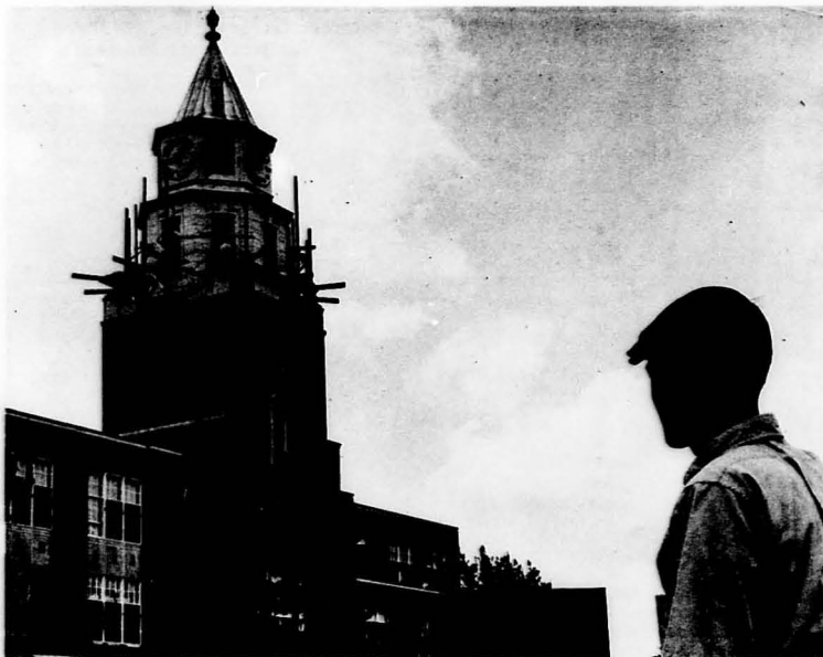
TIME FOR REPAIRS—Workmen have erected scaffolding around the clock tower of the University school tower—not to correct the clock but to paint the tower and repair the brickwork.
