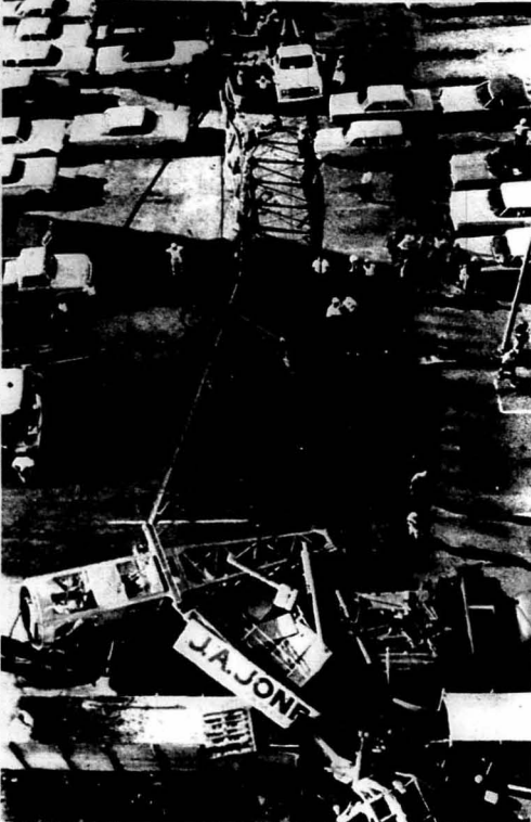
CRANE FALLS FROM BUILDING --This view from the top of a building under construction shows a crane that toppled down ten stories recently. The crane operator who rode the crane to the ground is in critical condition. One end of the crane struck the back end of an automobile in the parking lot across the street sending its three girl occupants to the hospital. The crane was atop a new addition to the General Telephone company in Tampa, Fla. (AP Photo)
