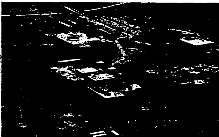
AERIAL VIEW SHOWS CONSTRUCT 'N PROGRESS ON FIVE EDWARDSVILLE CAMPUS BUILDINGS.
