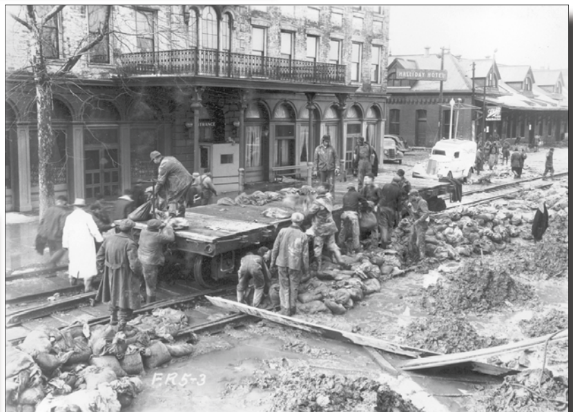
WPA men loading sand bags on railroad car for bulkhead on Ohio levee. Halliday Hotel [and Illinois Central Depot] in background. January 27, 1937.
