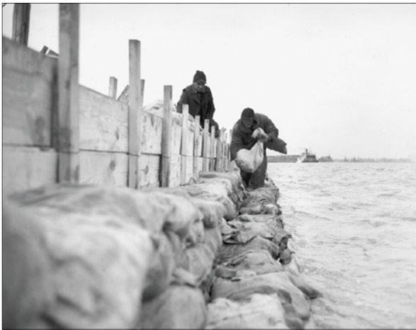
WORKERS ON THE LEVEE AT CAIRO, Ill. —Two of the army of relief workers, shipped in by the government, busy piling sandbags on the levee, here, to hold off the rising Ohio River. Warriors of a city under siege, these men have so far been successful in their efforts to keep back the mighty river.
