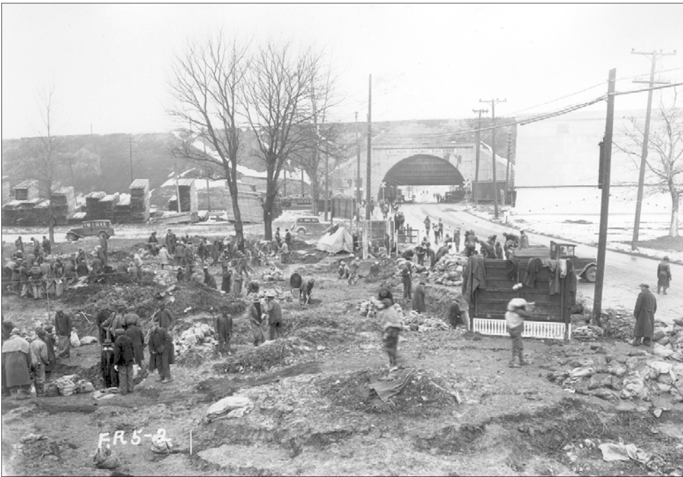
Works Progress Administration (WPA) men filling sand bags at entrance of subway on Route 51, Cairo, looking north. January 27, 1937.
