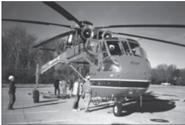
One of eighteen helicopters maintained by Erickson Air-Crane, Olga is nearly in constant use for the installation of HVAC equipment for its capabilities of lift and precision placement.
