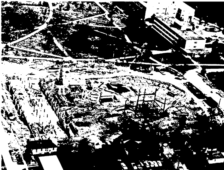
WORK PROGRESSES - This is an aerial view of the new Classroom Building at SIU, and shows progress on the new structure near Morris Library. Photo by Richard Prillaman.
