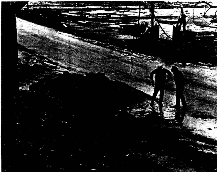
WHERE MAIN BROKE—The water supply to campus was disrupted Tuesday morning by a break in the main near the city filtration plant
