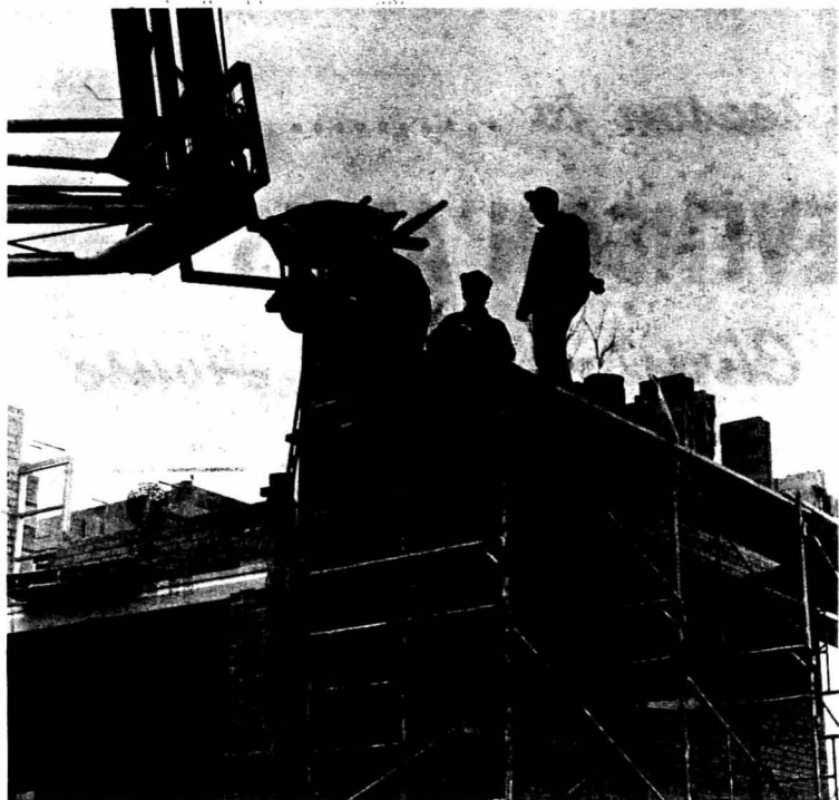
RISKY BUSINESS —A crane lifts a wheelbarrow to bricklayers atop the new Baptist Student Center at Mill Street and Campus Drive as construction on the building progresses. Work on the $850,000 structure is scheduled to be completed in September. The Center will have dormitory spaces for 300 students, both men and women, and provide cafeteria service. Also in the building will be a chapel room, recreation hall, library, classrooms and offices.
