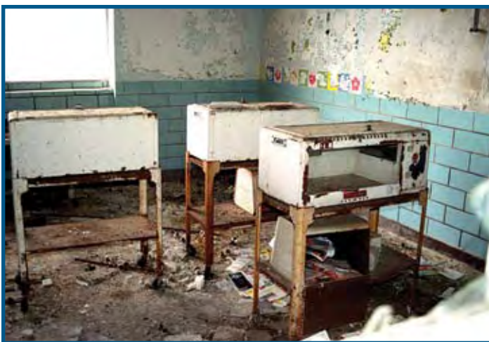
▲ Equipment sits in decay at Cairo's abandoned hospital. Photo courtesy The Cairo Project.
