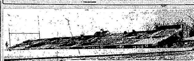
ABOVE: Newly completed S. I. N. U. stadium where 1500 seats are now being installed. Next Thursday it will be the scene of a parade, choruses, and folk dances when the Musical Festival is presented here. Formal dedication of the stadium which was built by W. P. A. labor and has a seating capacity of more than 6000 persons, will probably be held next fall.
