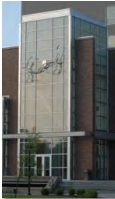
Figure 2-3. Morris Library renovation detail.
