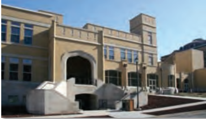
Figure 2-5. Altgeld Hall, new addition, October, 2004.
