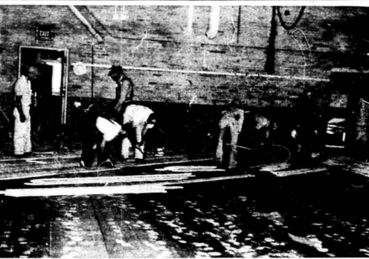
A $12,000 "FLOOR-LIFTING" job on Southern's gymnasium has reached the quarter mark.
